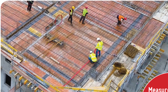
Installation of 3DSensor within reinforced concrete slab
