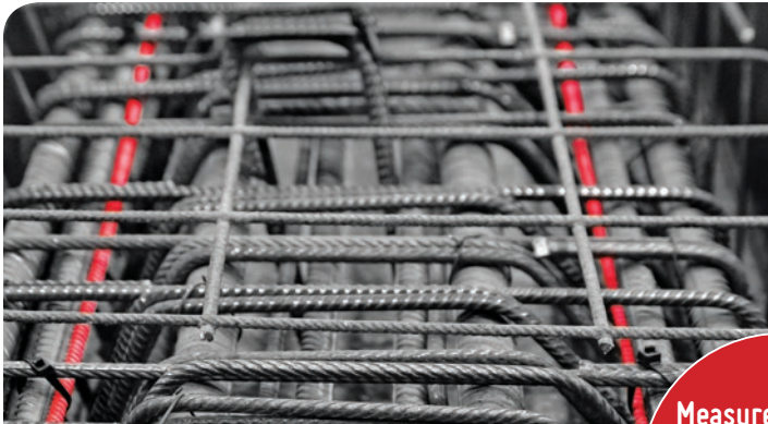
Prestressed concrete beam with EpsilonRebar
