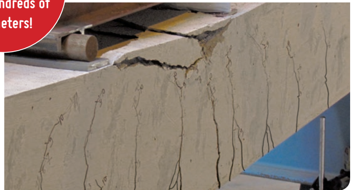
Crack measurements by EpsilonSensor during bending tests
