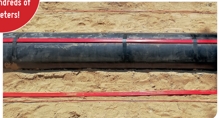
Application of 3DSensor along a gas pipeline
