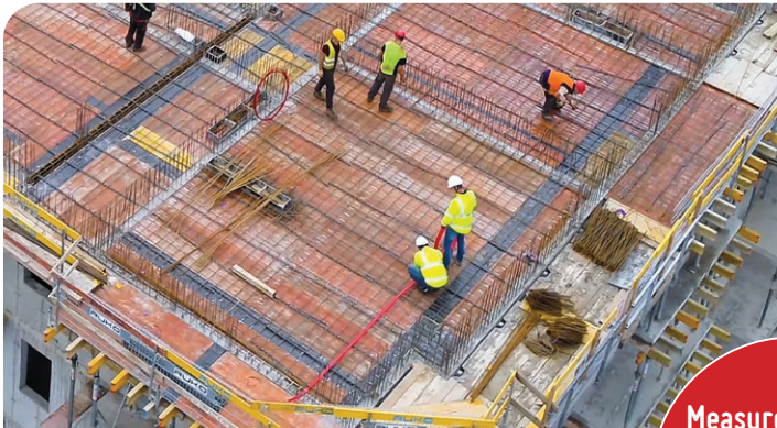
Installation of 3DSensor within reinforced concrete slab
